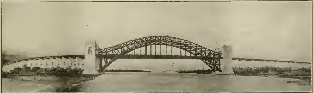
HELL GATE BRIDGE AND APPROACHES OF THE NEW YORK CONNECTING RAILROAD.
